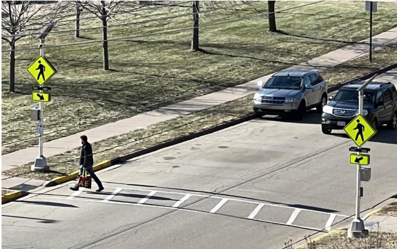
Rectangular Rapid Flashing Beacons Example in Platteville, WI
