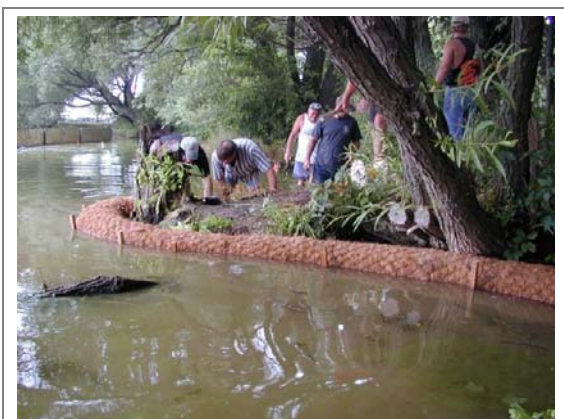
Photograph 3.3-2. Example of a bio-log restoration site.
