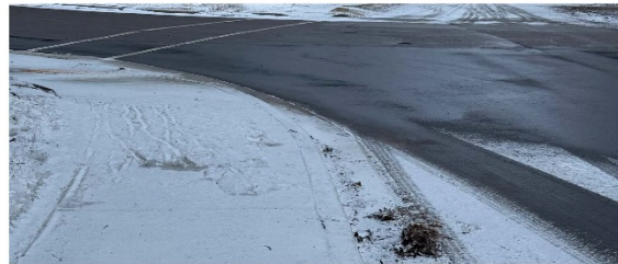
Image 8: Snowy tire tracks show vehicles cutting the corner as tight as possible, then swinging out.
